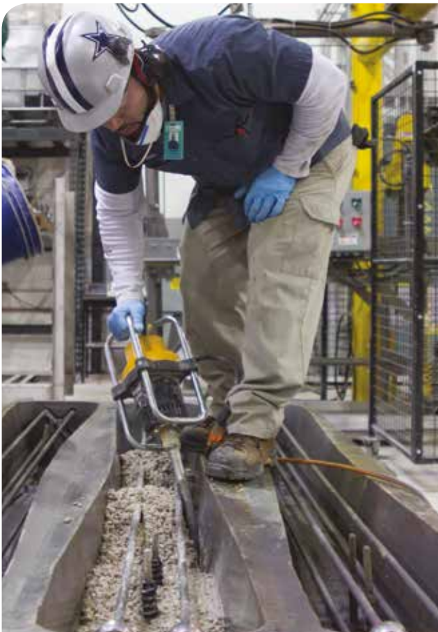
Figure 4. Vibration casting of Solidia Concrete in a railroad sleeper ('tie') mold.
